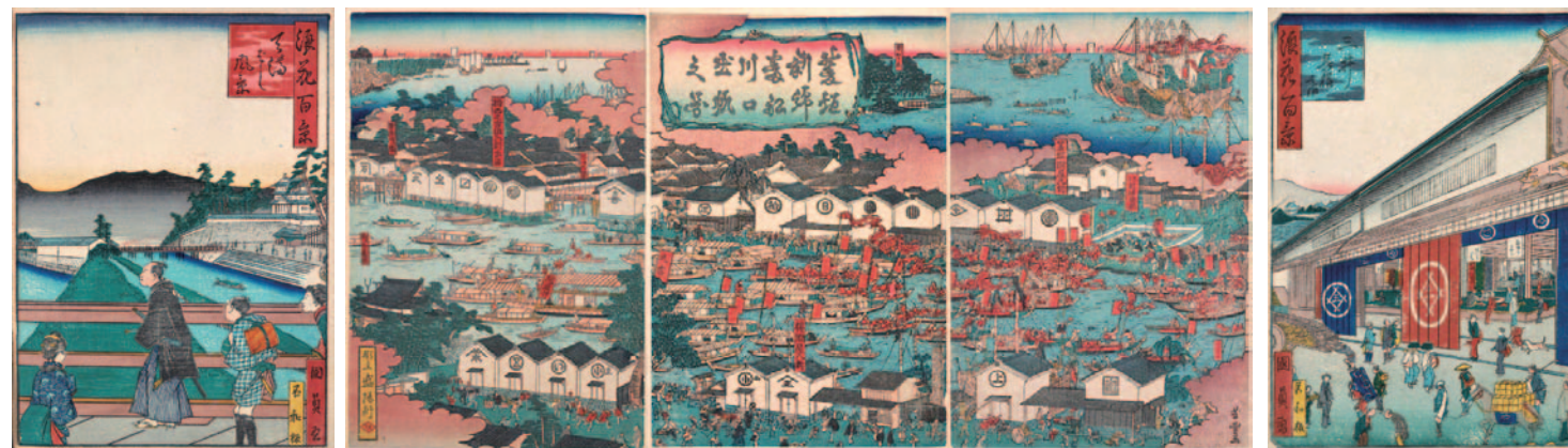
① View of Temma Bridge
